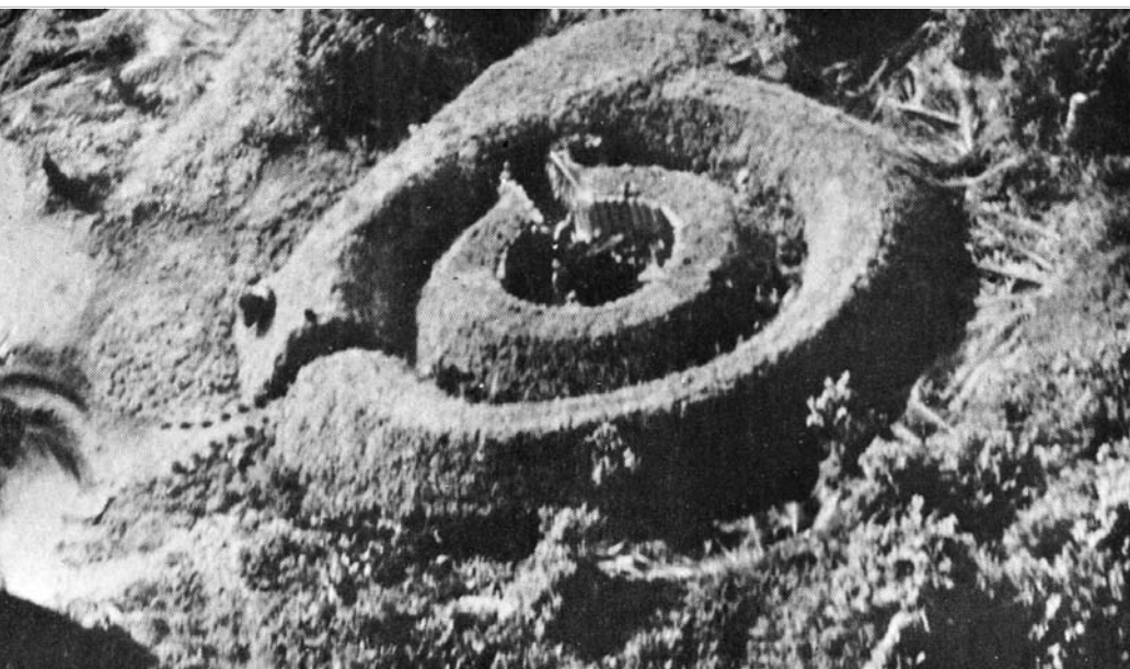
This riveting aerial photograph taken during the raid on Kavieng on February 15, 1944, depicts a newly completed earthen revetment protecting a Japanese dual-barrel 25mm anti-aircraft gun emplacement. These weapons posed a significant threat to low-flying B-25s on bombing and strafing runs.
